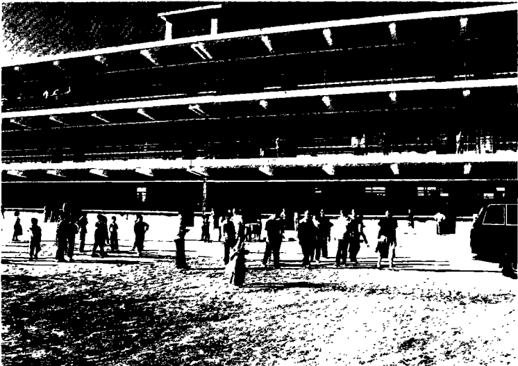
A new primary school is built to a high standard in Xiji, Tongxian.
